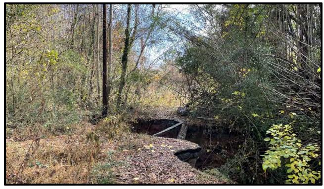
Photo 24 - the site from Fletcher Street; the creek has washed out the culvert
